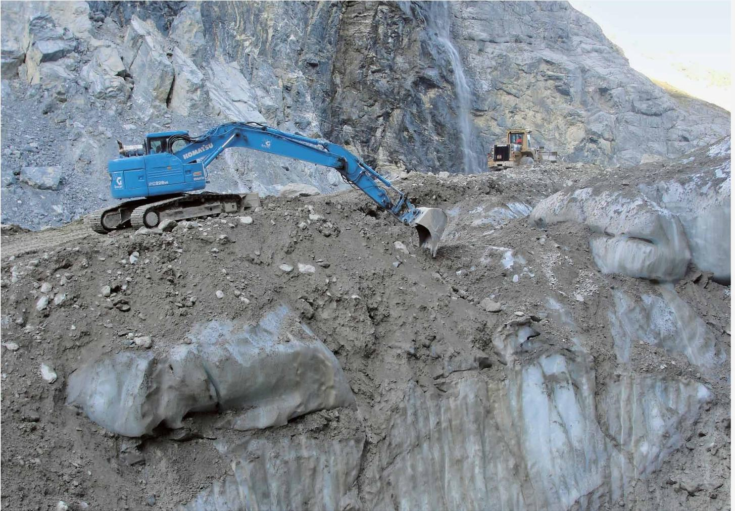
Construction work on the Unterer Grindelwald Glacier (Canton Bern) on 7 October 2009: The glacier has retreated to a huge extent in the last 150 years. In 2005 a lake formed for the first time on its surface. In 2009 a drainage tunnel was built in order to avert the danger of a glacial lake outburst flood.
